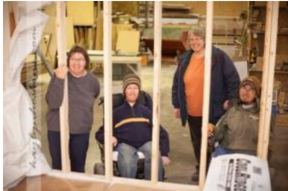
Sue, Josh, Kathy Finholt, and Jacob check out their new home while under construction at All-American Homes in Dyersville, IA
